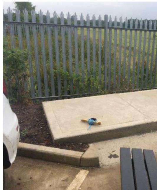
**Figure 13: Plinth for the Battery Units**
