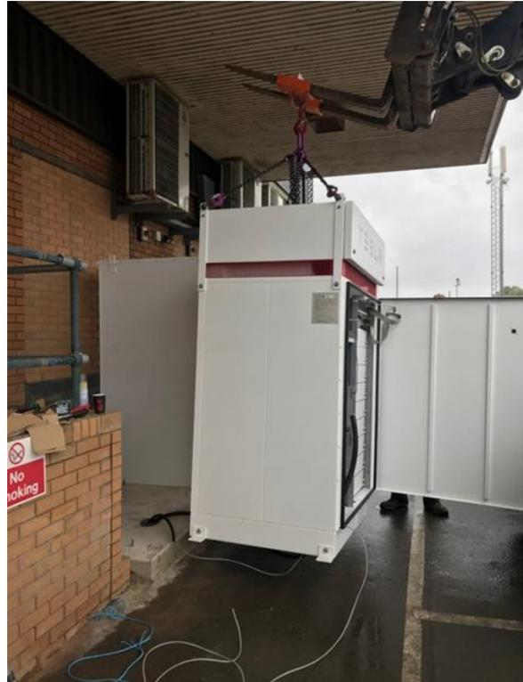
**Figure 11: Battery Units Lifted by Crane**
