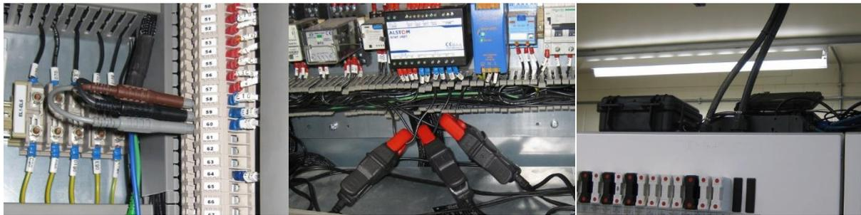
Figure 2-1 – Pilot PQ monitor installation at Meaford C. From left to right: connections in to VT secondary wiring; current clamps around CT secondary wiring; Envoy communications hub and PM7000 PQ monitor installed on top of switchgear.
