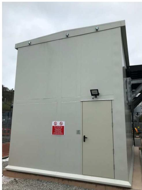
**Figure 2-14: Transformer Noise Enclosure**
