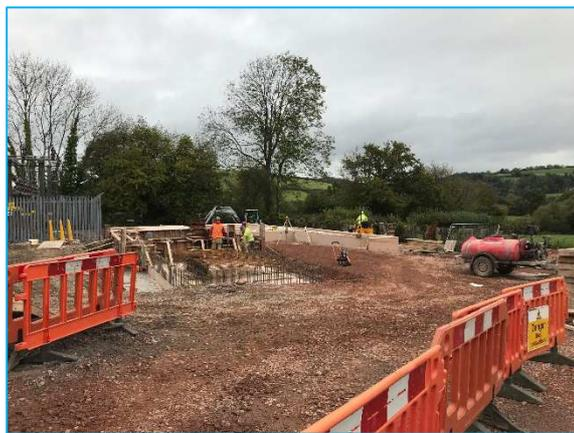
Figure 2-25: Installation of plinths
