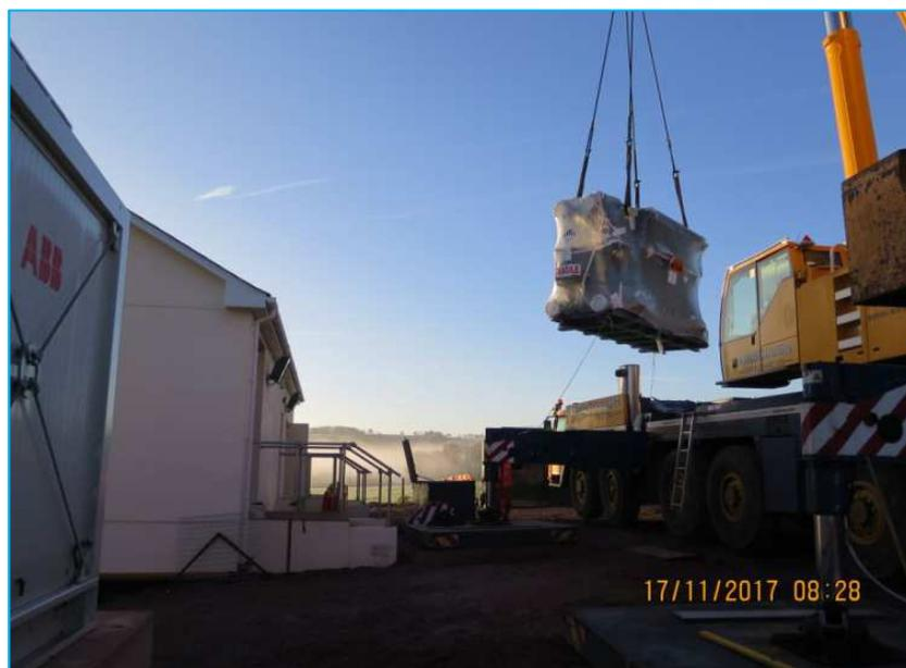
Figure 2-28: Delivery of transformer
