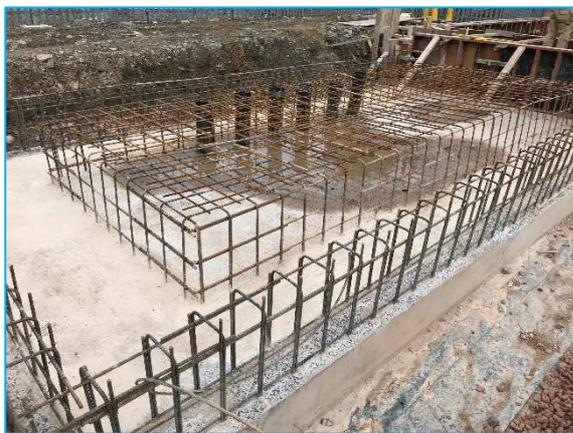
Figure 2-24: Rebar for transformer plinth
