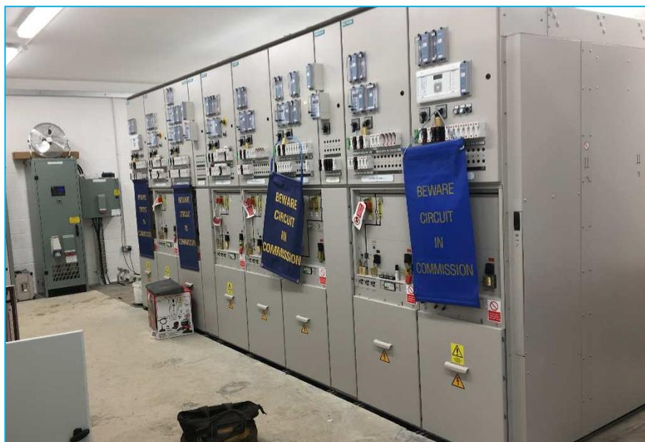
Figure 2-26: 33kV switchboard being commissioned
