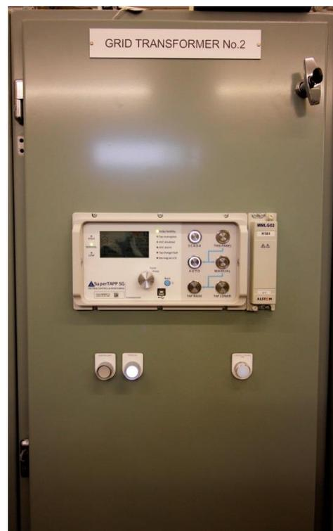
Figure 10-4: Detail of GT2 SuperTAPP SG Installation
