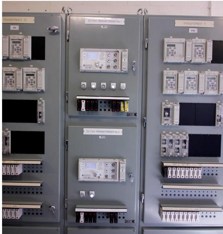
Figure 42-1: Replacement Front Doors Containing SuperTAPP SG Relays
