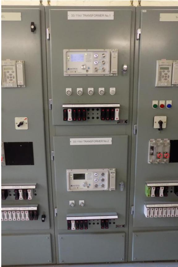
**Figure 38-1: Replacement Front Doors containing SuperTAPP SG**
