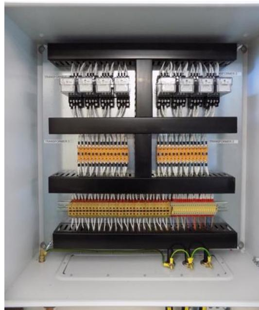
Figure 2-19: MicroTAPP SVO Control Panel Wiring at Waterlake Primary Substation
