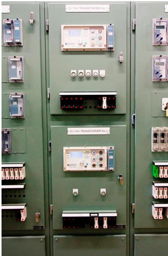
Figure 2-18: SuperTAPP SG Relay Install at Colley Lane Primary Substation
