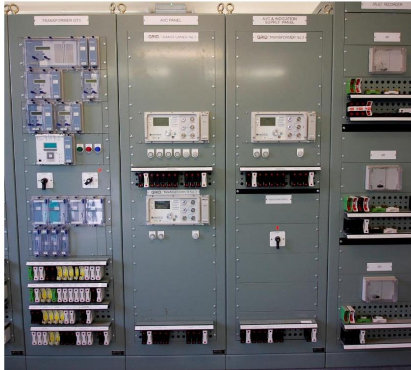
Figure 14-1: GT1, GT2 and GT3 SuperTAPP SG Installation
