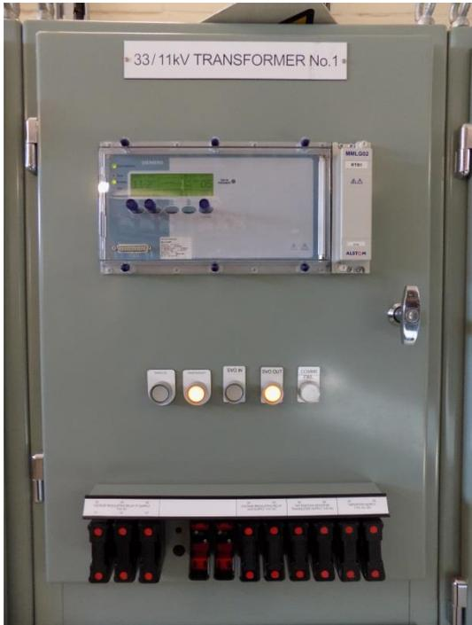
Figure 70-1: SVO Control Modifications to T1 Panel
