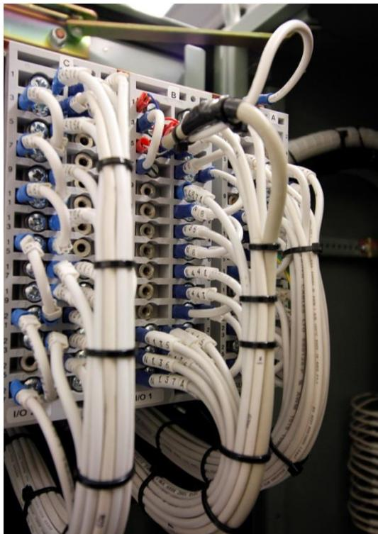
Figure 34-3: Wiring to back of MicroTAPP relay
