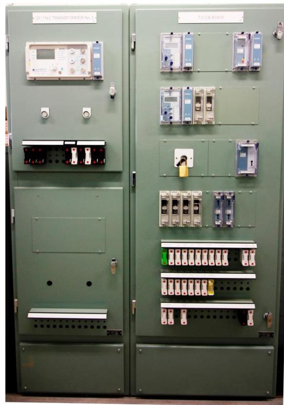
Figure 18-2: T3 SuperTAPP SG Installation
