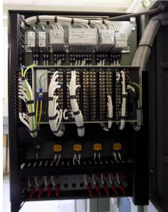
**Figure 38-2: Rear of Front Door with SVO Controls**
