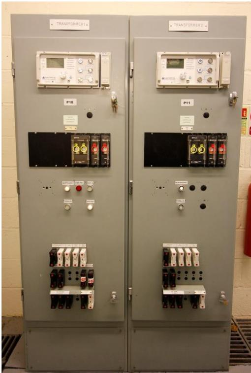
Figure 46-1: T1 and T2 Modified Tap Change Panels
