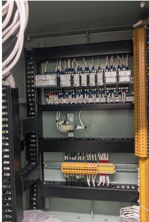
Figure 62-3: T1 Panel Internal Compartment
