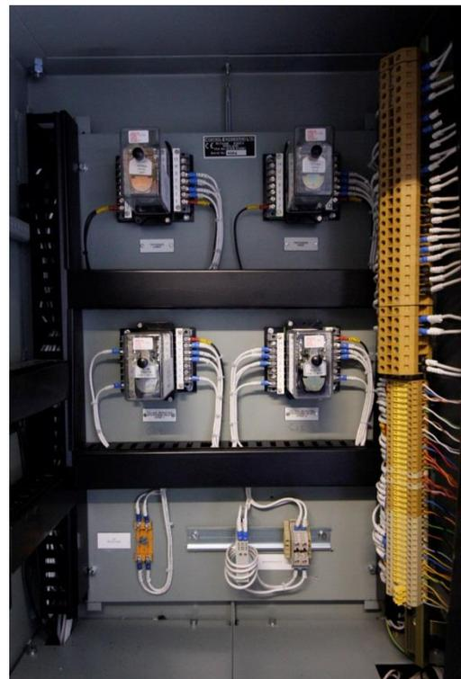
Figure 42-3: Internal Auxiliary Relays for T1
