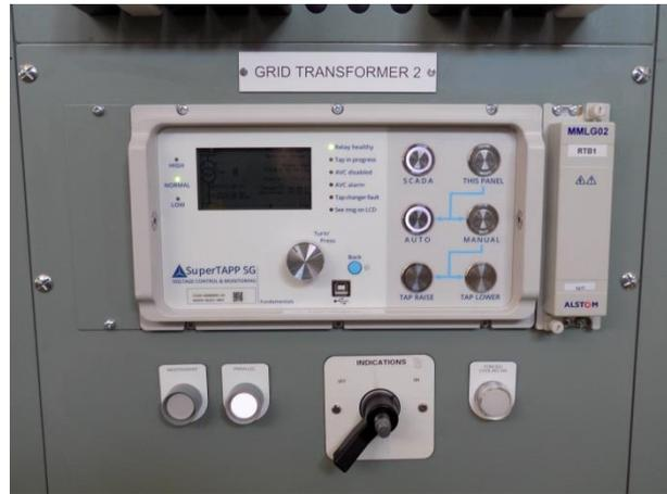
Figure 50-2: GT2 SuperTAPP relay and Controls
