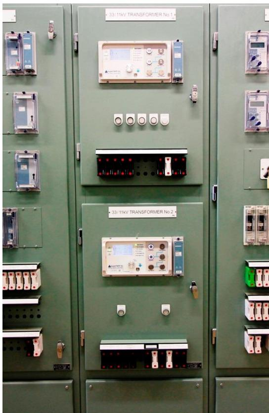
Figure 18-1: T1 and T2 SuperTAPP SG Installation
