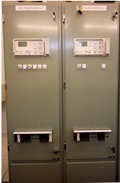
Figure 10-1: GT1 and GT2 SuperTAPP SG Installation
