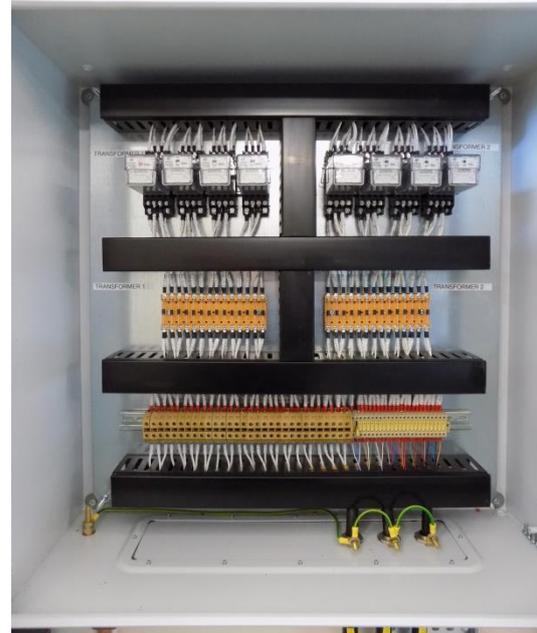
Figure 70-2: SVO Control Panel Internals
