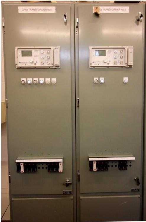
Figure 2-21: SuperTAPP SG Relay Install at Bowhays Cross BSP
