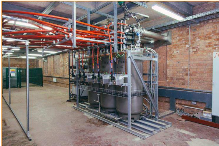
Figure 7-11: Bournville RSFCL shown in its final position at site
