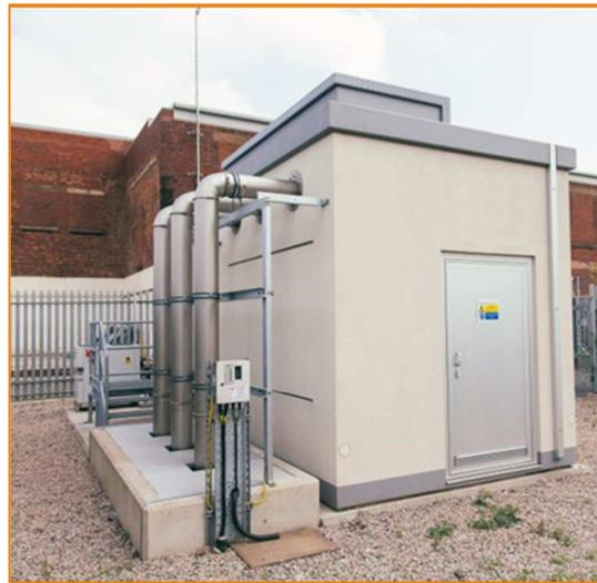
Figure 7-10: Chester Street RSFCL positioned and installed at site
