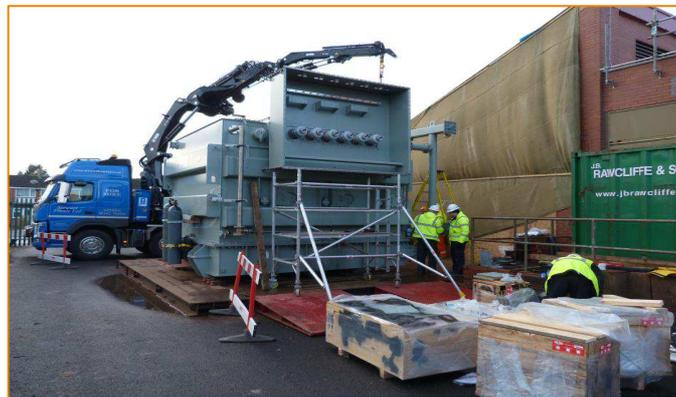
Figure 7-9: Castle Bromwich FCL being prepared for skidding into the spare transformer bay
