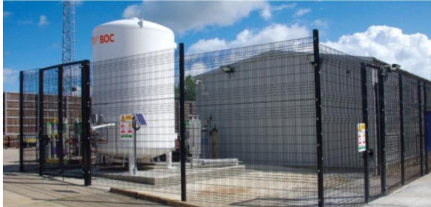
Figure 4.17: Outdoor secure liquid nitrogen storage [35]
