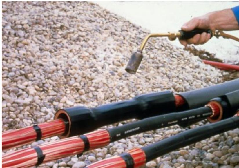
Figure 5.3: Raychem heat shrink cable joint
