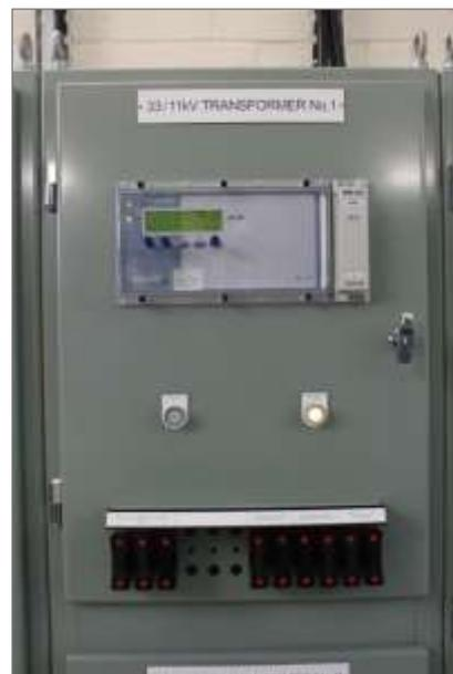
Figure 2-8: MicroTAPP AVC Relay
