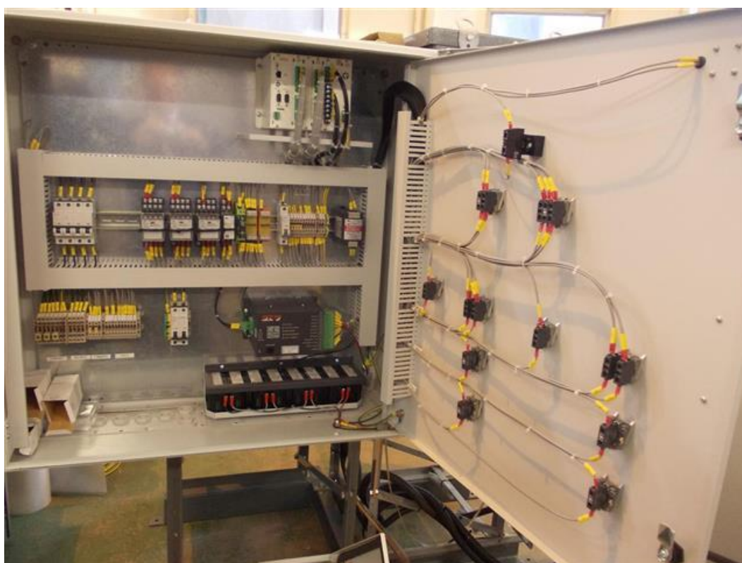
Figure 4 CCP (Internal Wiring)
