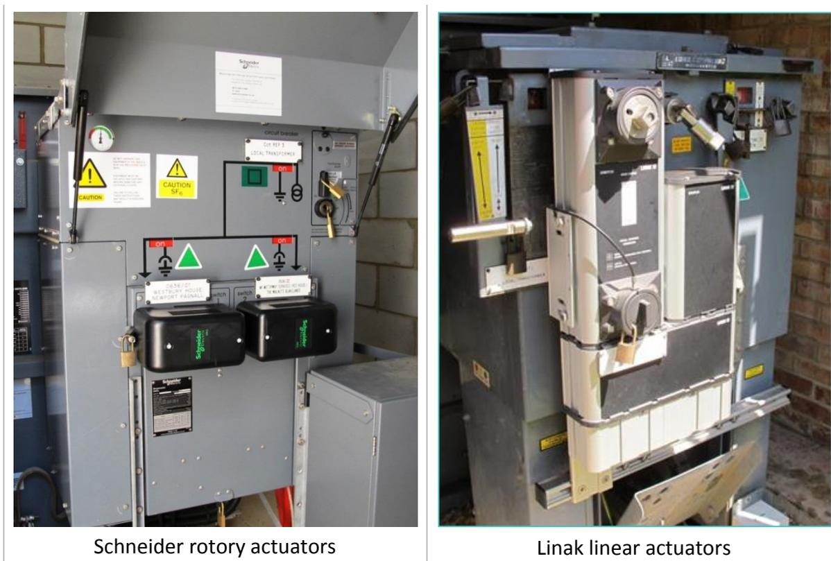
Figure 3 : Installed switchgear actuators.
