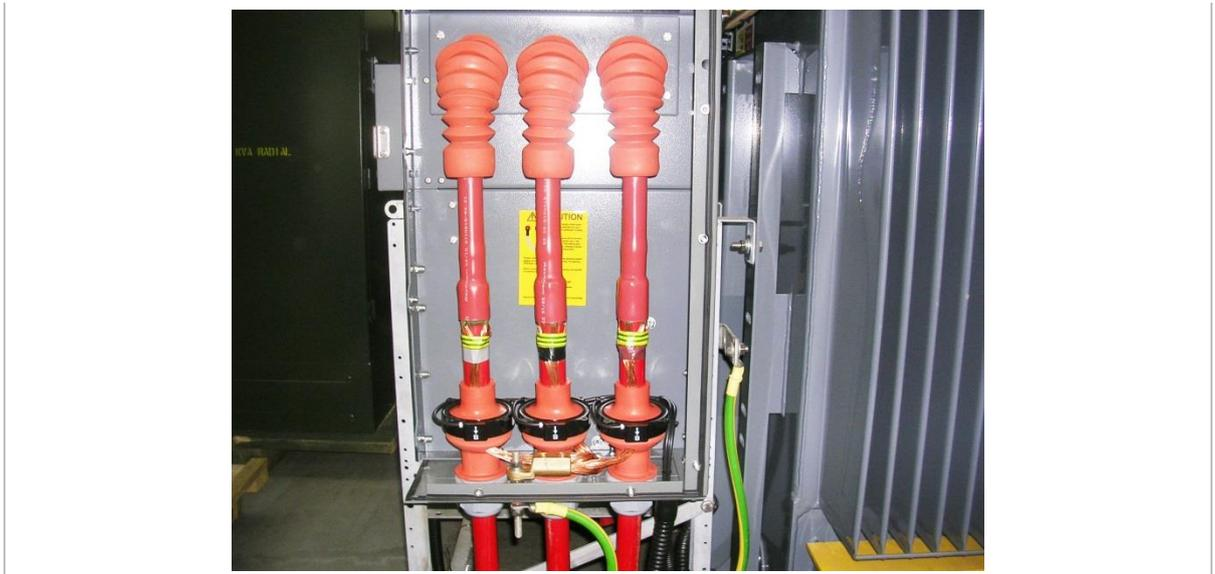
Figure 4 : Installed switchgear CT's.
