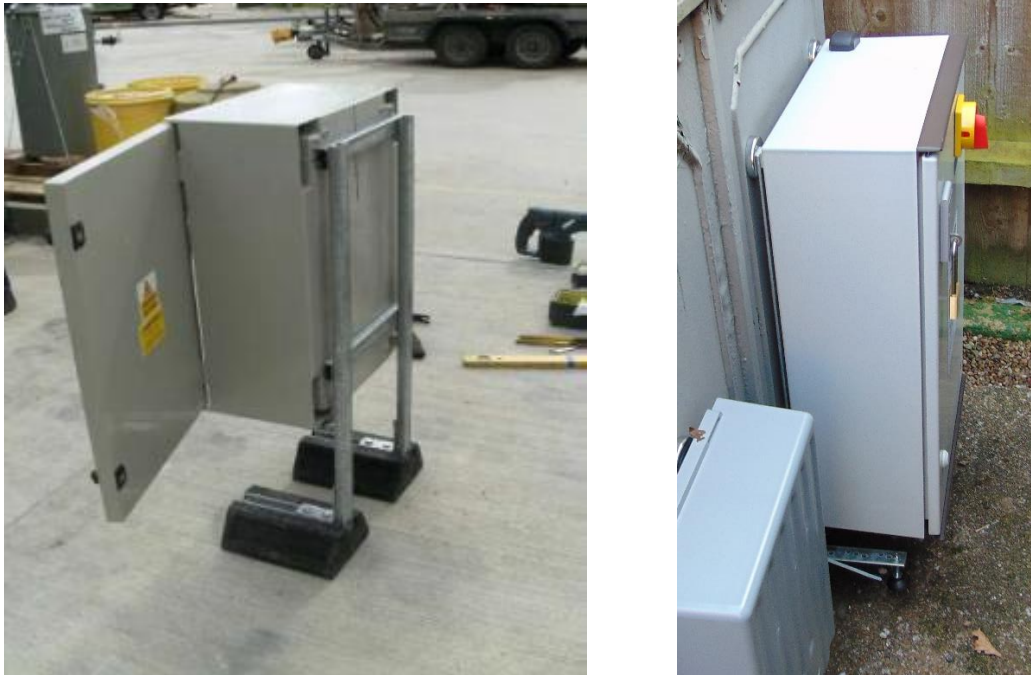
Figure 12: Examples of frame used to ground mount an enclosure
