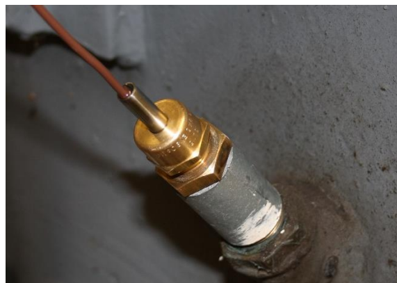
Figure 8: Example transformer oil pocket and test cap, including thermal probe
