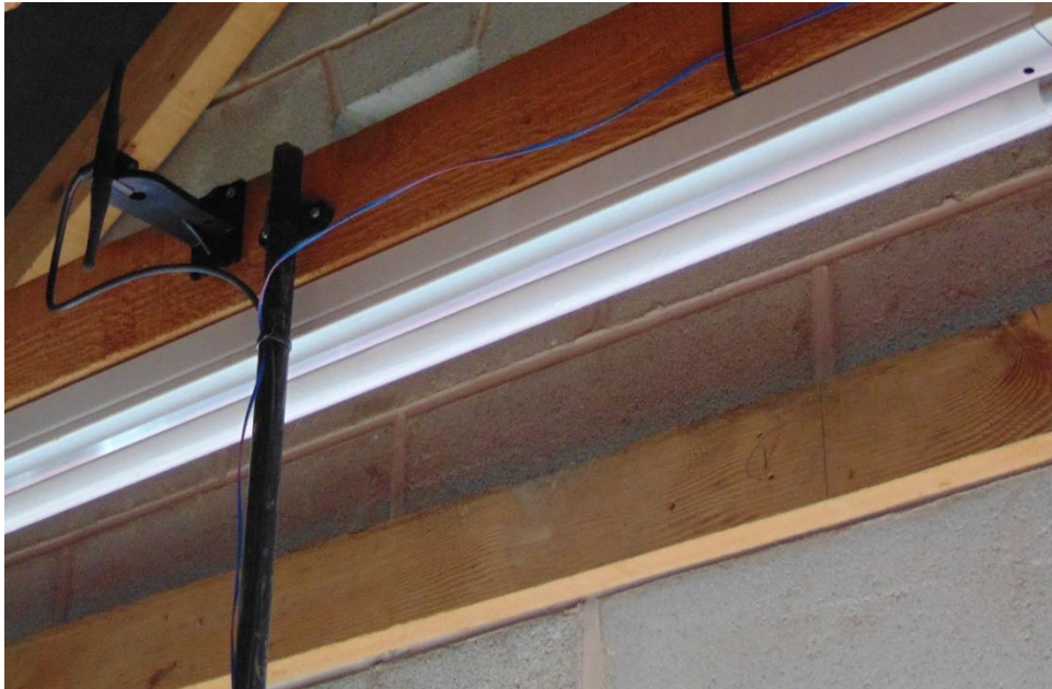
Figure 29: Mounting the mobile network antenna
