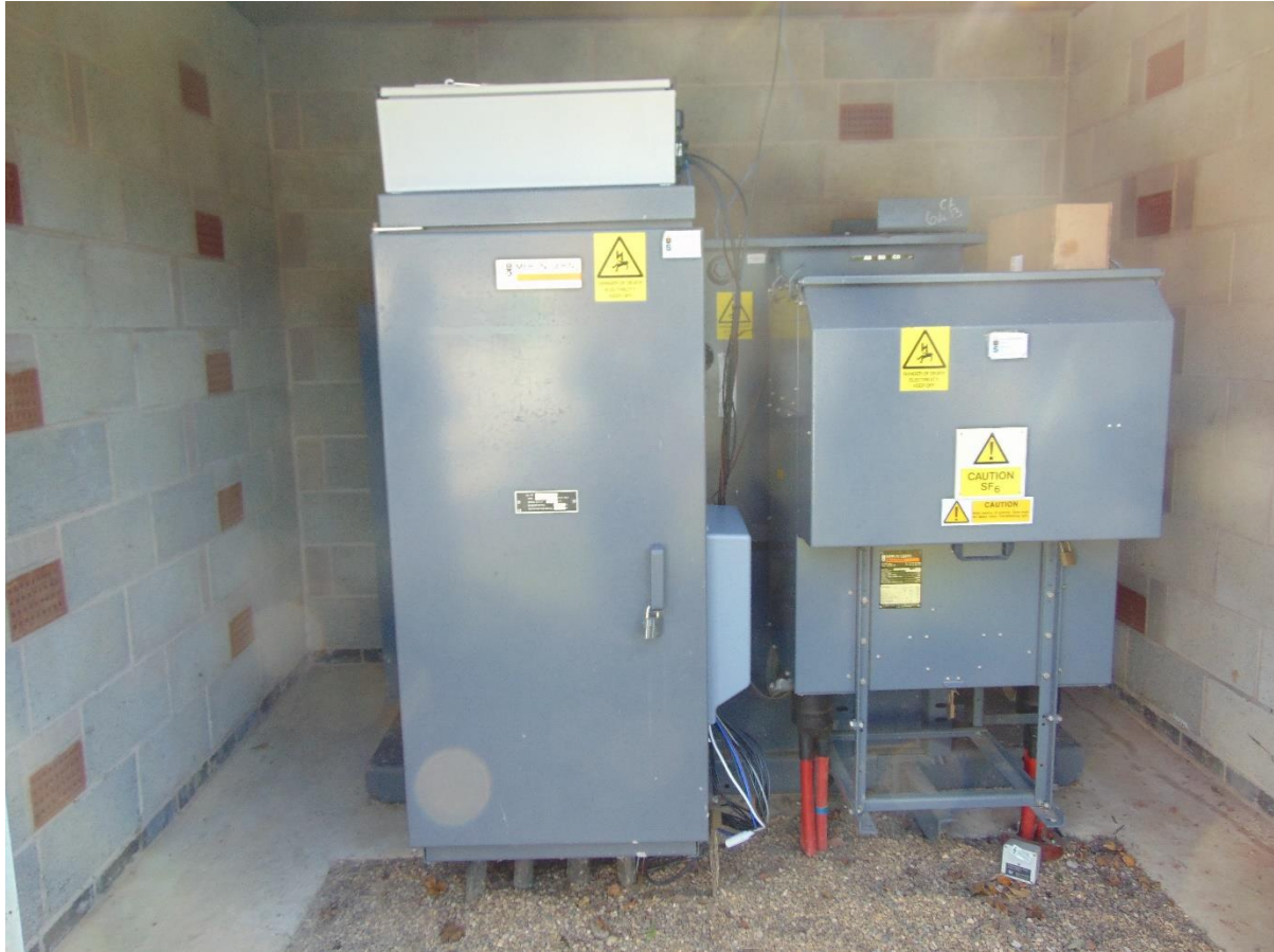
Figure 13: Space on top of a package substation arrangement
