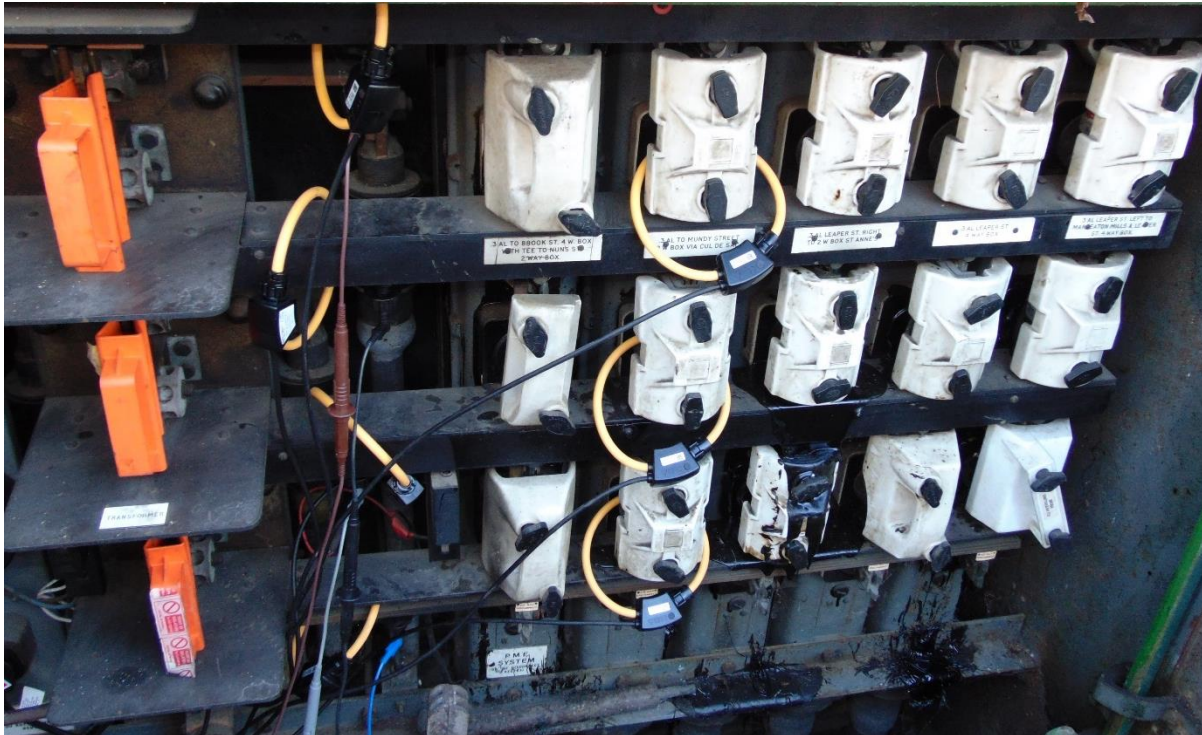
Figure 24: LV Busbar Monitoring
