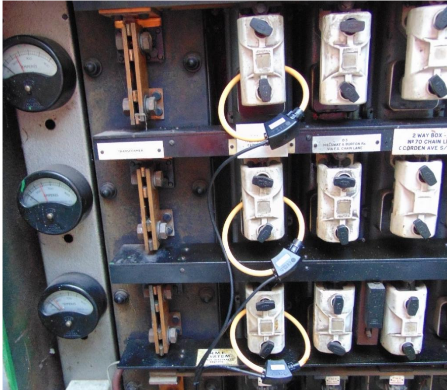
Figure 22: Flexible Rogowski Coils installed around fuse carriers
