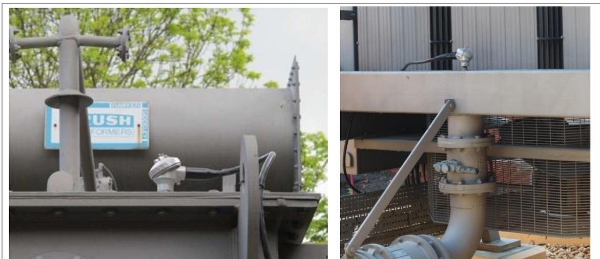
Figure 5 : Illustration of top of tank and bottom of cooler oil temperature sensor
