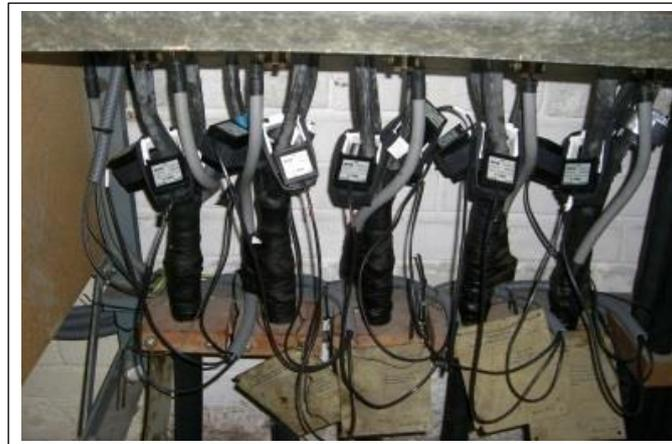
Figure 3 Substation Sensors
