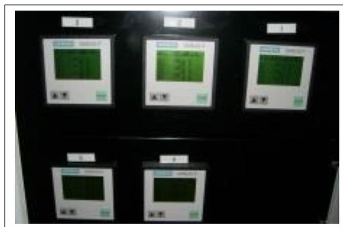
Figure 2 Substation monitoring meters
