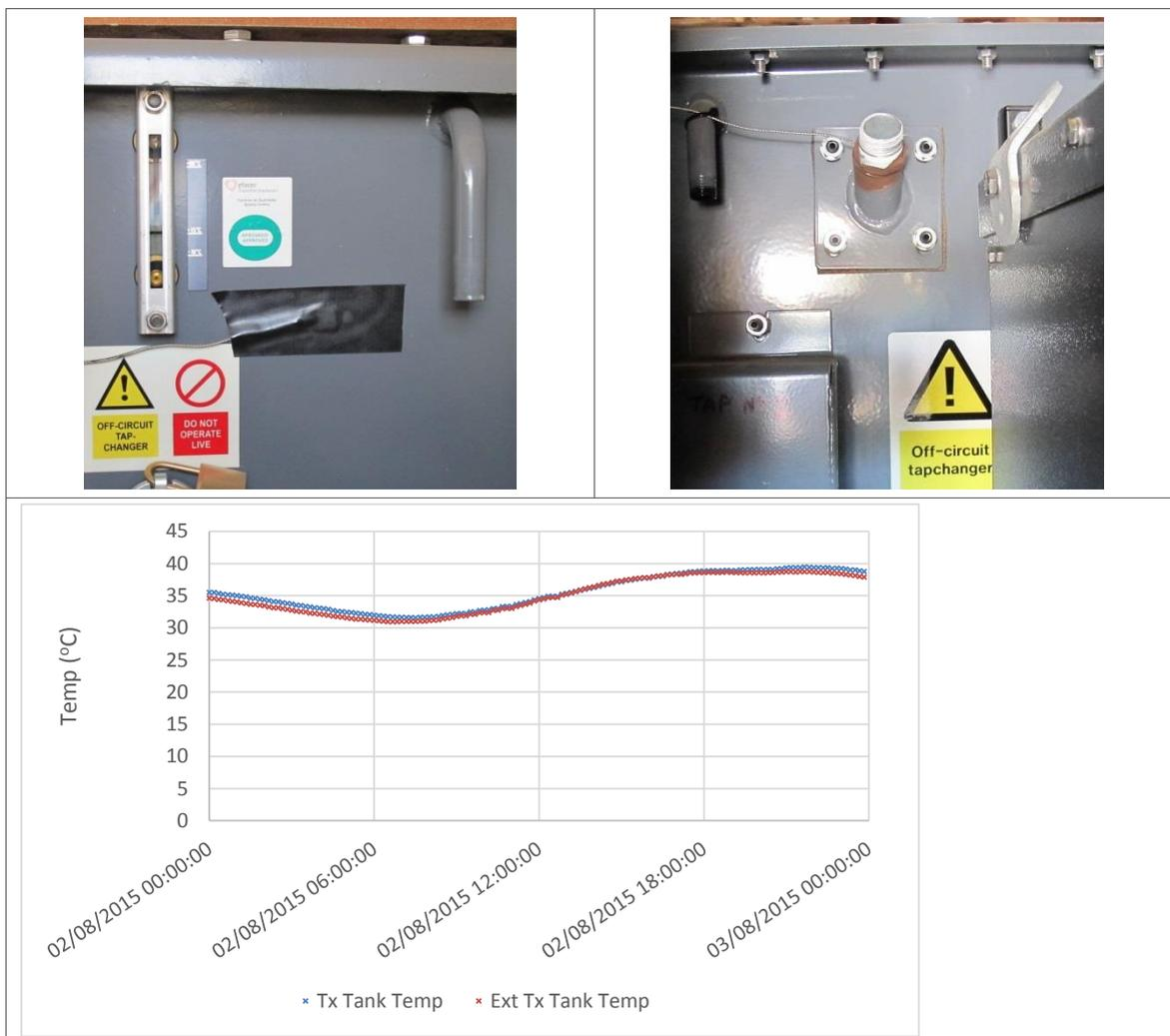
**Figure 6: Illustration of tank shim temperature measurement, thermometer pocket temperature measurement, and coincidence of measured values from a well-positioned external tank and thermometer pocket measurement positions.**
