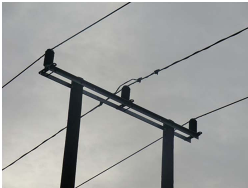
Figure 15 – Rebuilt line with fibre wrap
