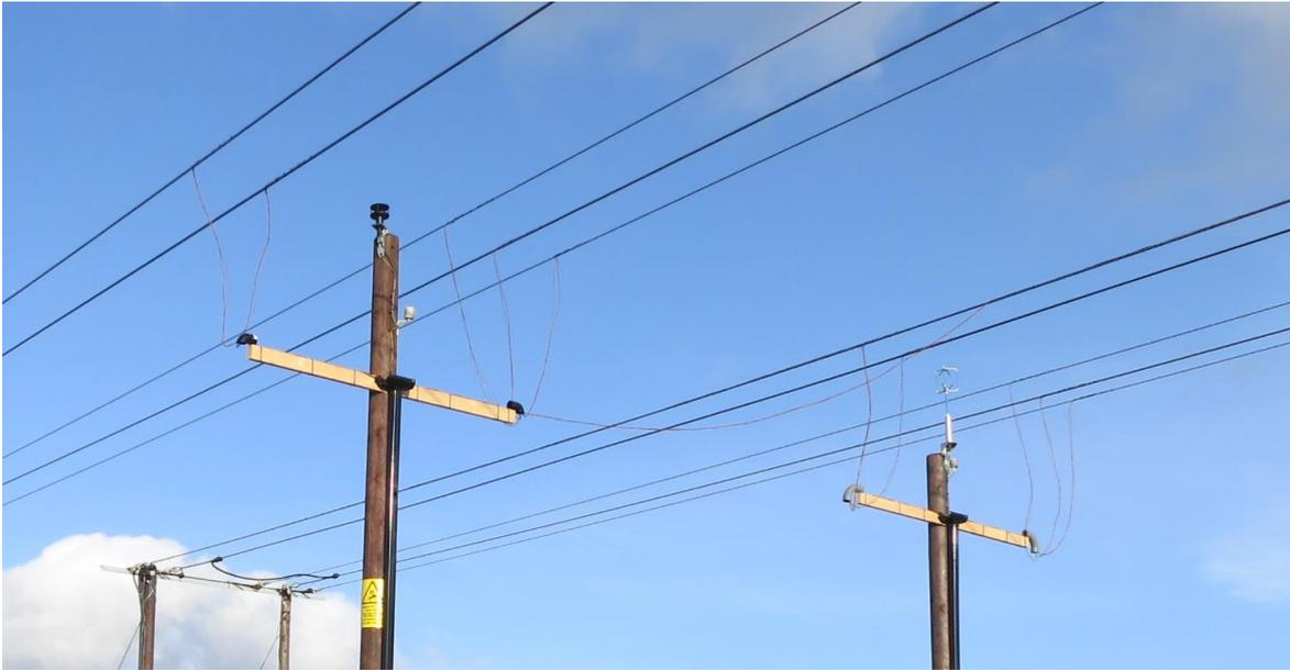
**Figure 6** Weather monitoring equipment installed on freestanding intermediate wood poles
