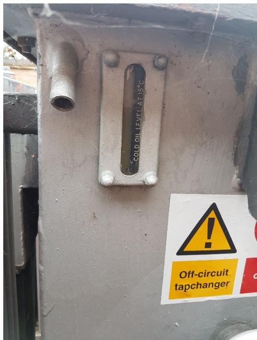
Fig. 1.1 : A typical pole-mounted transformer showing the head-space vent
