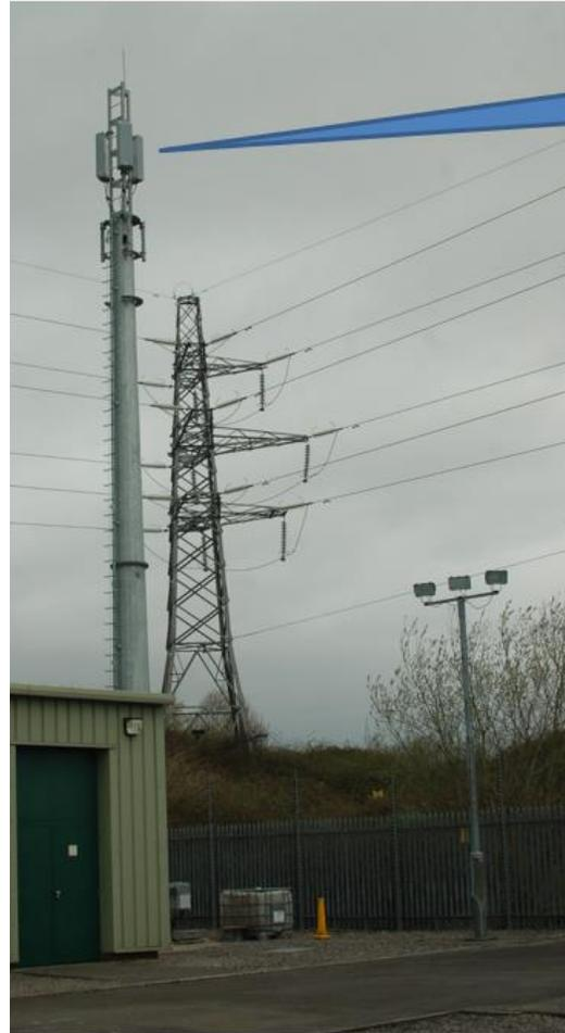
Tri-sector 400 MHz eLTE base station mast at Portishead Bulk Supply Point (132kV/33kV)
