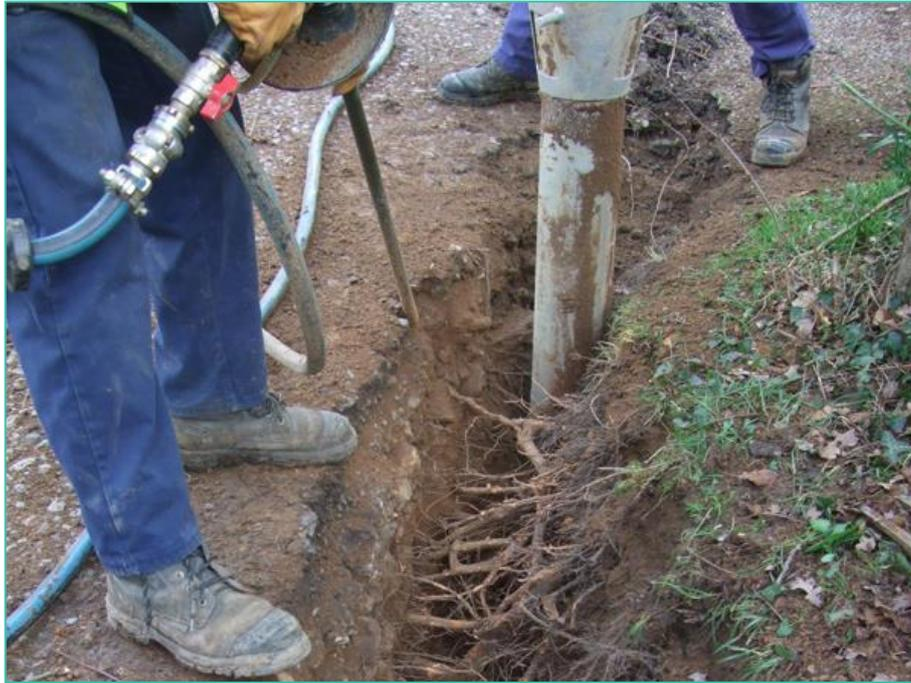
Figure 2-6 Illustration of vacuum excavation method
