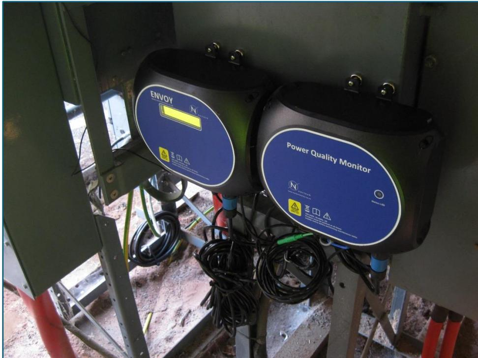
*Figure 5-40: Plug & play PQ monitor installation at an 11 kV distribution substation*
