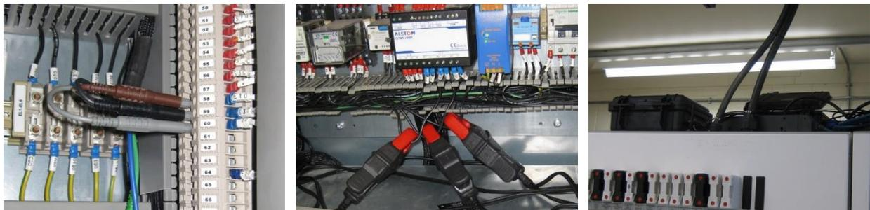
Figure 5-18: Pilot PQ monitor installation at Meaford C. From left to right: connections in to VT secondary wiring; current clamps around CT secondary wiring; Envoy communications hub and PM7000 PQ monitor installed on top of switchgear.
