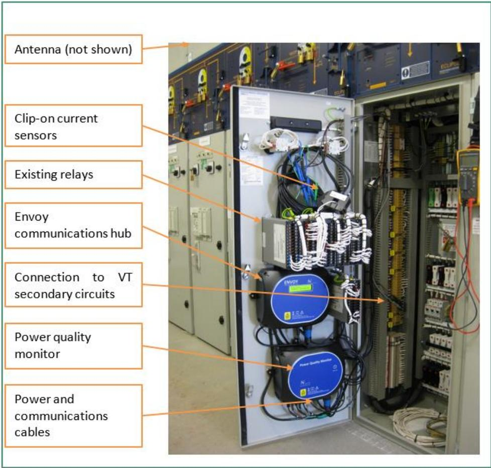
Figure 5-39: Example plug & play PQ monitor installation
