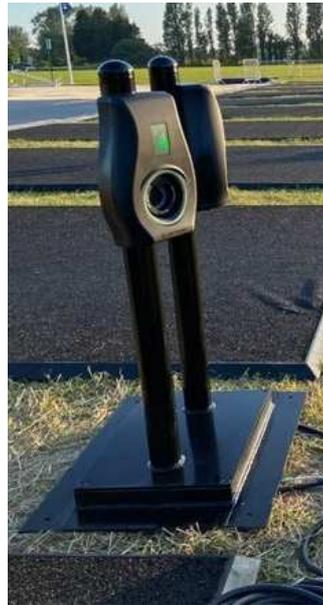
**Figure 5-2 Photograph of proposed EVCP arrangement for temporary events**
