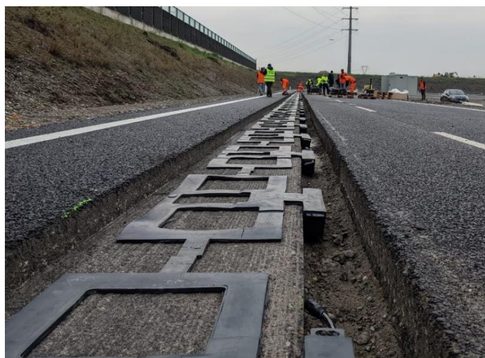
Figure 17: Photo from the ElectReon deployment in Italy in November 2021.
