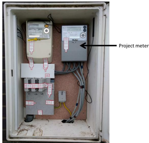
**Figure 8** Installed three-phase meter at commercial premises
