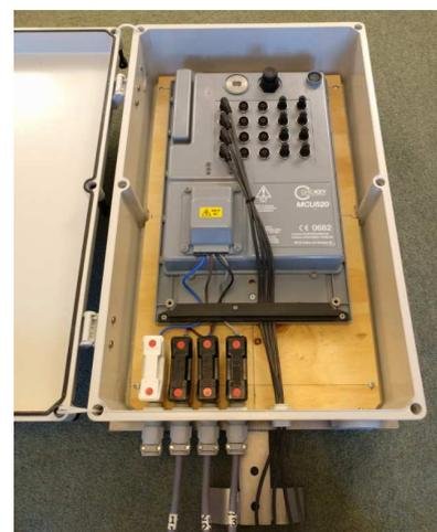
Internal arrangements of pole mounted transformer monitoring cabinet
