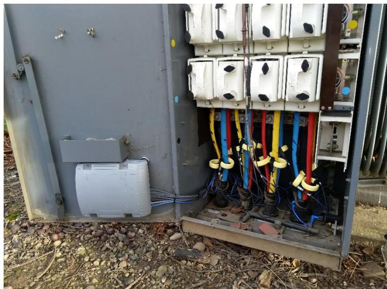
As it is unrealistic to generate these types of arc events in a laboratory or controlled conditions, WPD nominated various substations that were suspected to be active with pecking events for the distance to fault equipment to be fitted to.
