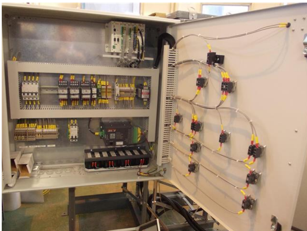
Figure 4 CCP (Internal Wiring)
