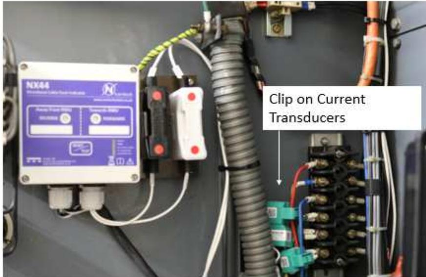
**Figure 5: Clip on variant of NX44 unit installed within a primary circuit breaker.**
