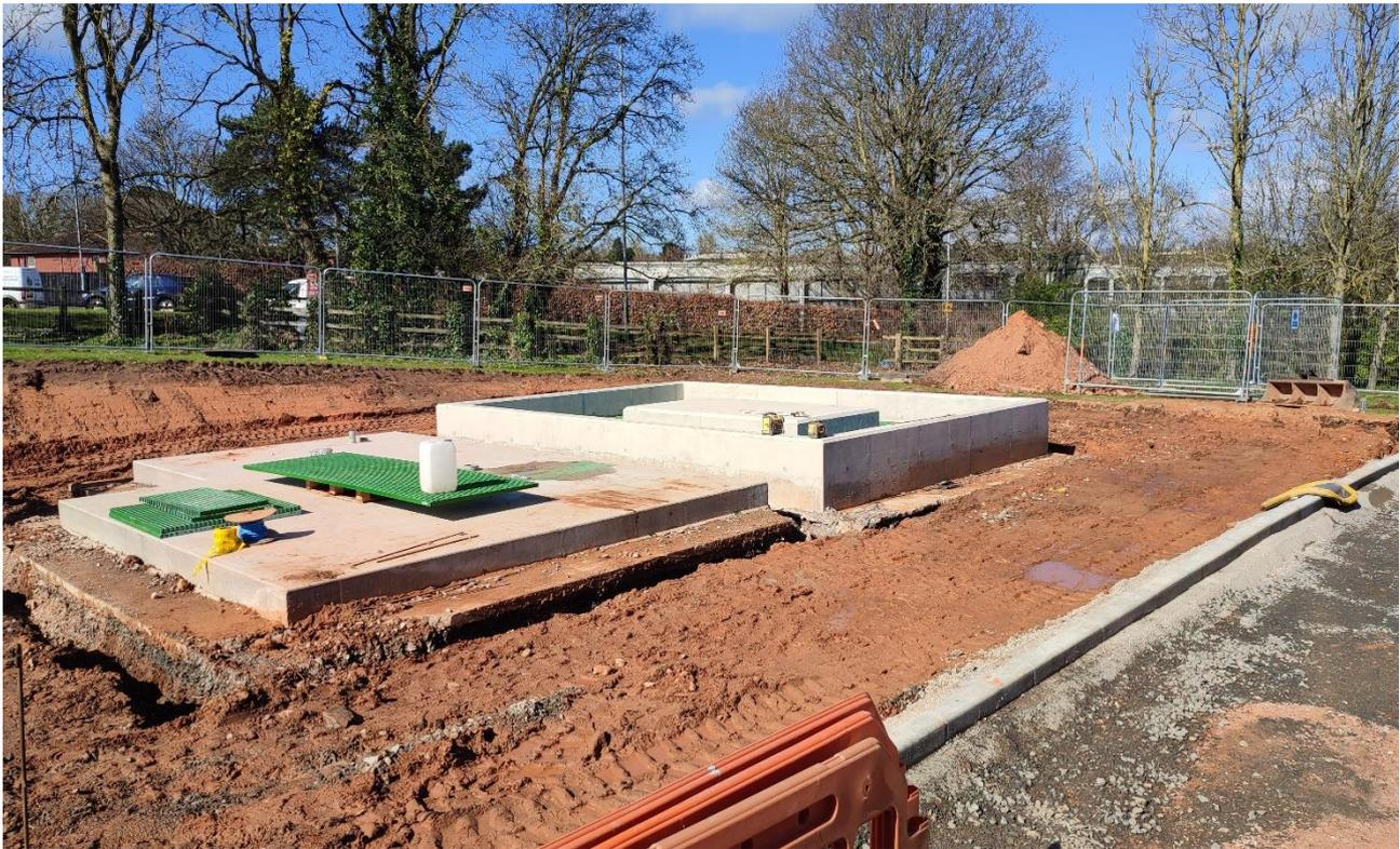
Figure 13 Plinths for switchroom container and transformer
