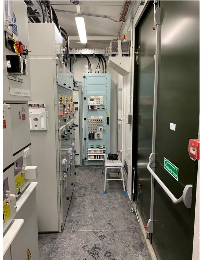
Figure 5 View of 11 kV switchgear
