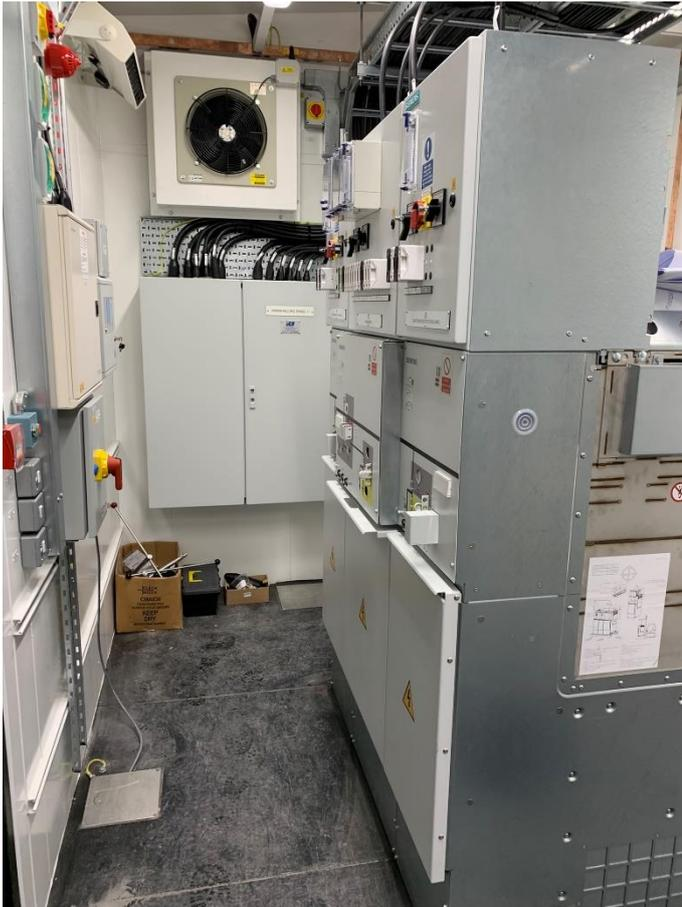
Figure 4 View of 33 kV switchgear
