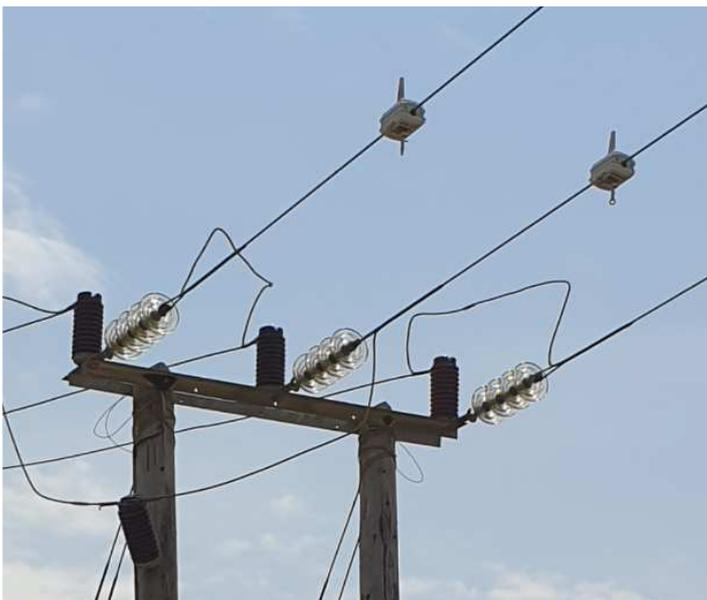
**Figure 5-1 MetySense 5000 sensor set on a feeder supplying St. Blazey 33/11kV substation**
