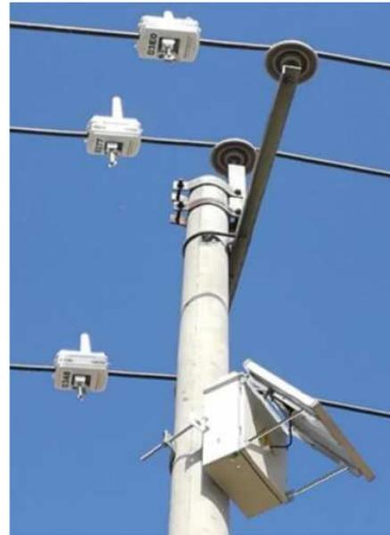
**Figure 5-2: Example of a pole mounted gateway unit**
