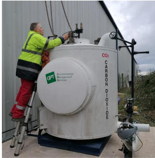
Figure 2 Liquid carbon dioxide storage tank
