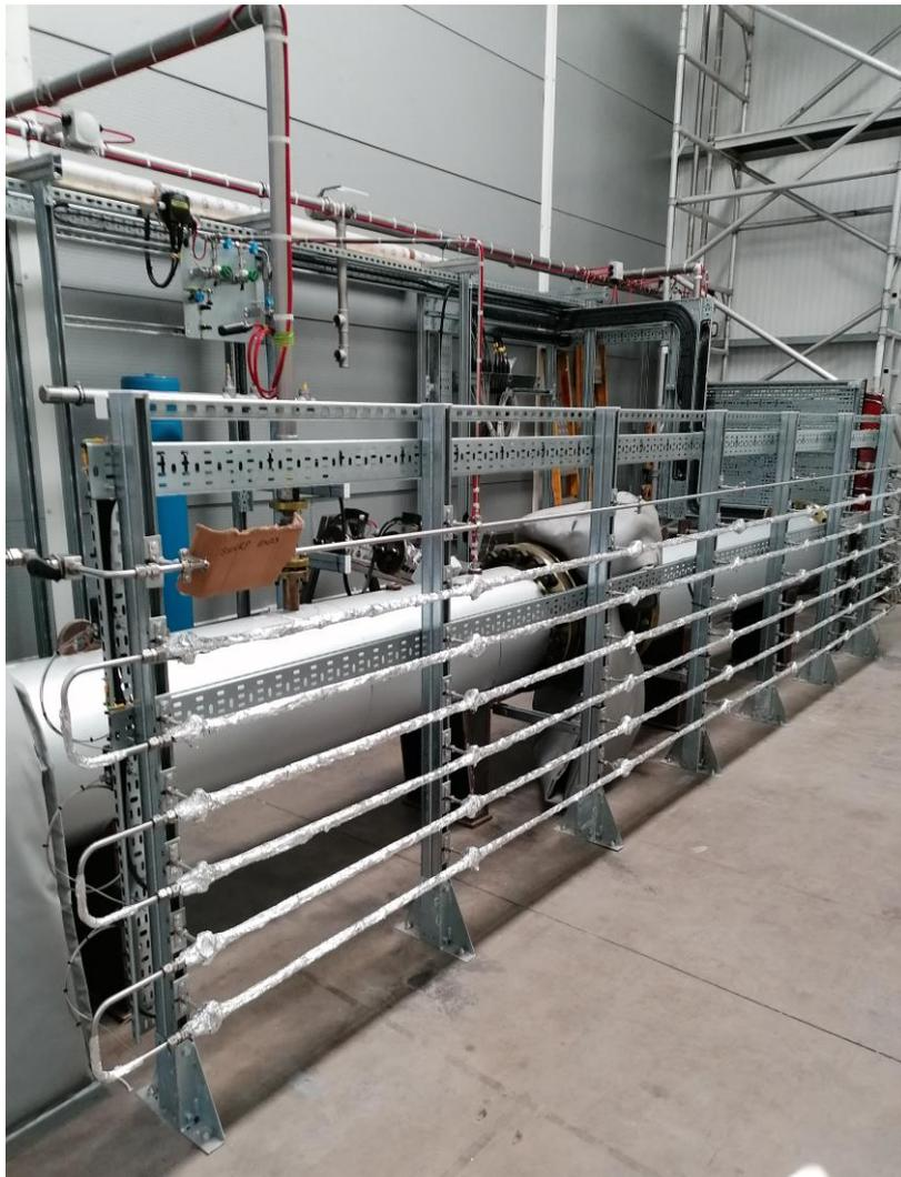
**Figure 6 Extraction System Heat Exchangers**
