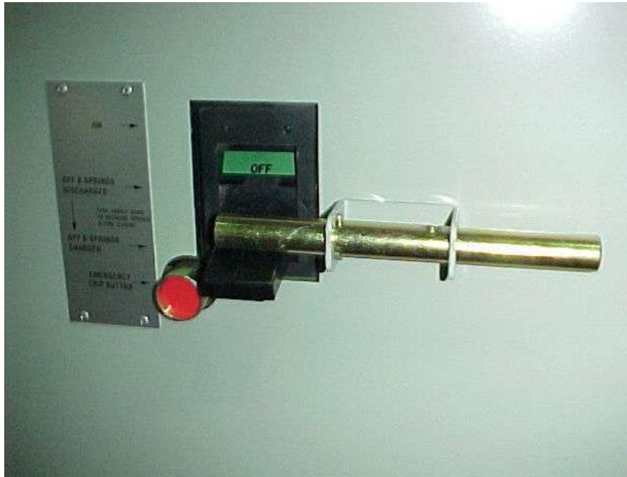
Figure B2 Metering MCCB Locking Arrangement
