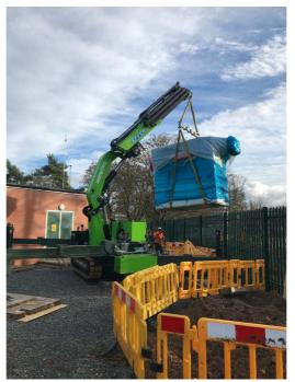
Figure 2-1 Crane offloading FCLi being onto the concrete foundation at UoW
