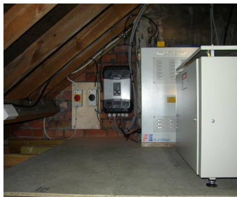
The completed Loft Installation
