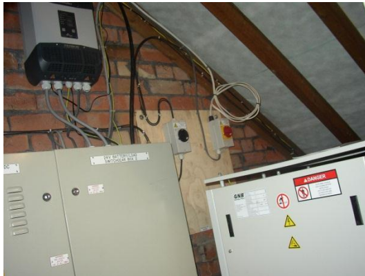
Figure 3 - The completed Loft Installation
