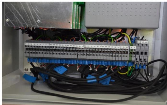
Figure 23: Rogowski coils wired into loom. (WPD)
