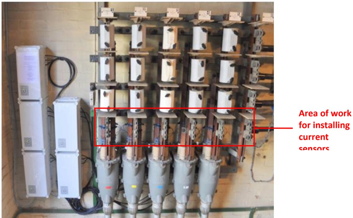
Figure 1: Area of work highlighted for Lucy B1 and B2 type board
