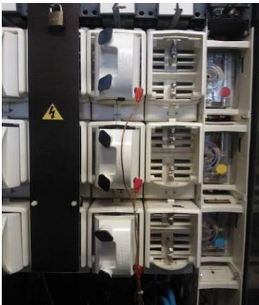
Fuse Carrier with red Auxiliary voltage plugs
