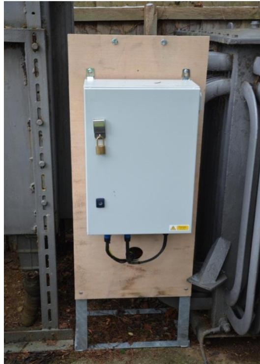
**Figure 2:** GMC i-Prosys metrology unit installed in outdoor substation. (WPD)
