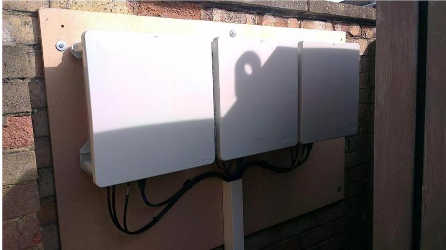
**Figure 20:** Ambient metrology units, one for each LV way. (WPD)
