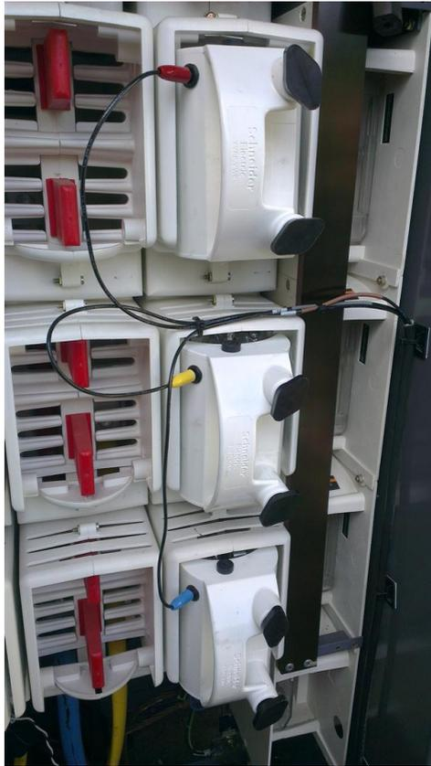
**Figure 11:** Modified fuse carrier handles installed on spare leg in pillar
