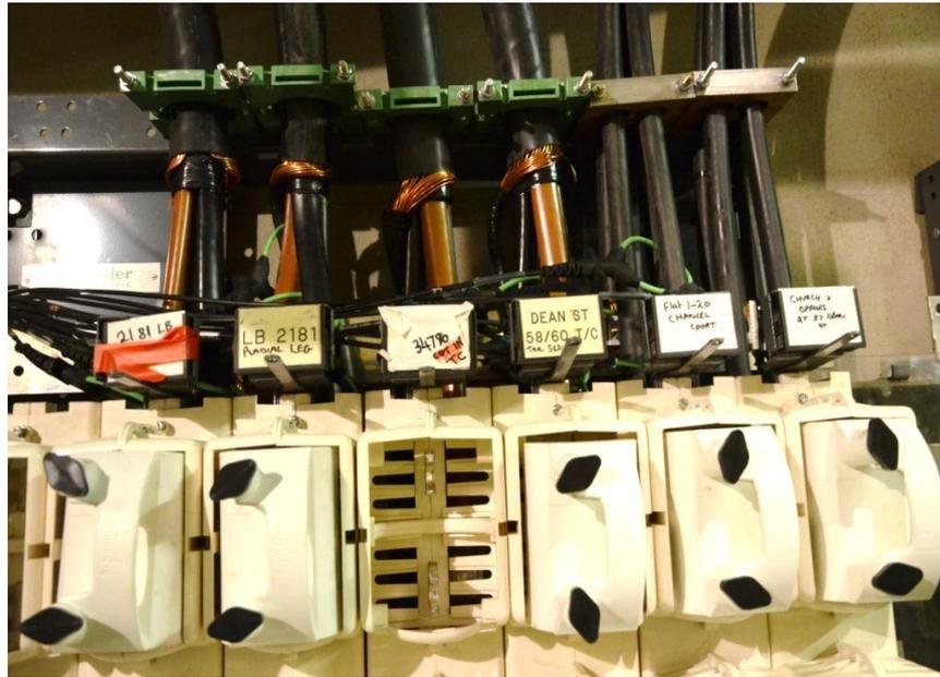
**Figure 3:** GMC i-Proslys Rogowski coils installed around tightly spaced cable cores.
