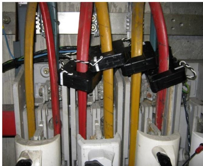
**Figure 19:** Ambient CTs around core conductors on an open LV board. (UKPN)
