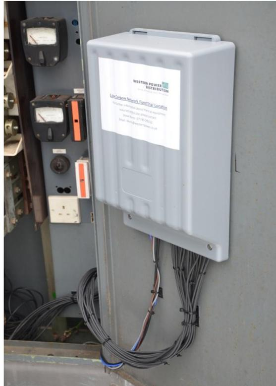
**Figure 5:** Sensor cables and voltage/power cables coming into the metrology unit (WPD).
