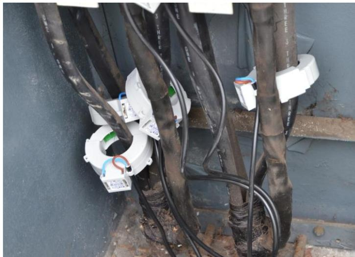
**Figure 12:** PowerSense split core CTs around LV phase cores (WPD).
