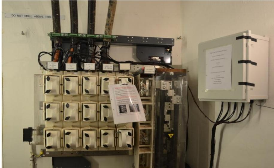
Figure 24: Haysys monitoring solution installed in substation. (UKPN)
