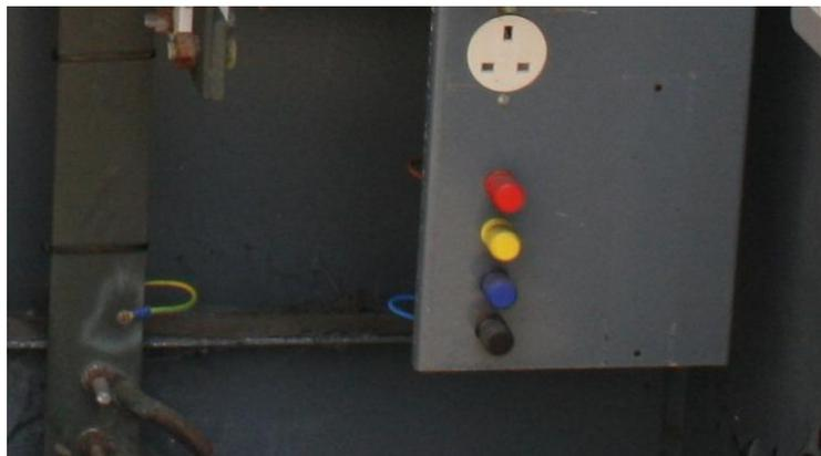
**Figure 7:** LV Cabinet with 3 phase test point
