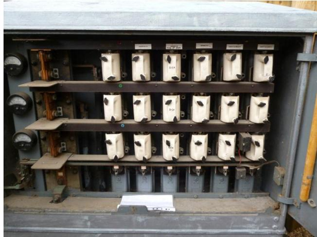
**Figure 4:** LV cast iron cabinet with compound filled tiered cable terminations.
