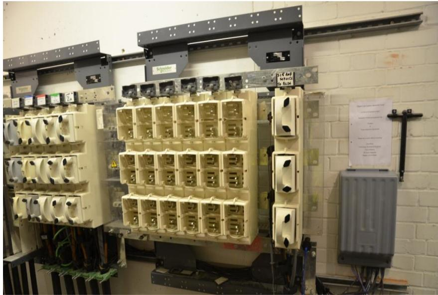
**Figure 6:** The GridKey MCU with the sensors and voltage leads connected. (UKPN)
