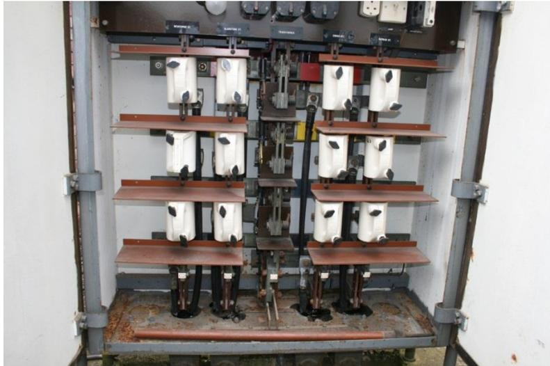
**Figure 8:** LV Cabinet with open busbar design
