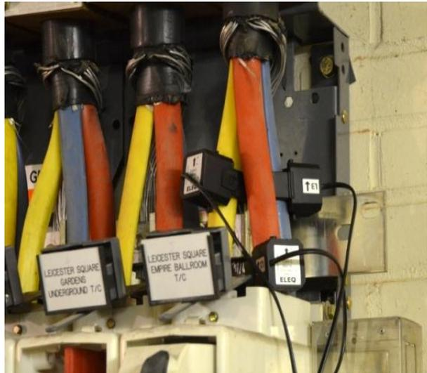
**Figure 27:** Locamation split core CTs around individual phase cores. (UKPN)
