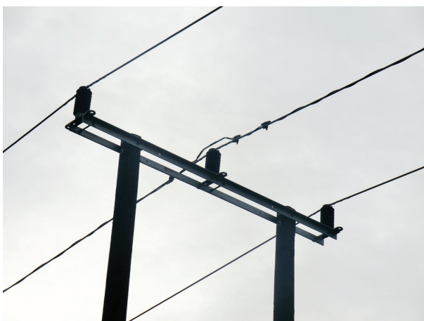
Figure 13 – Fibre wrapped OHL (middle conductor)
