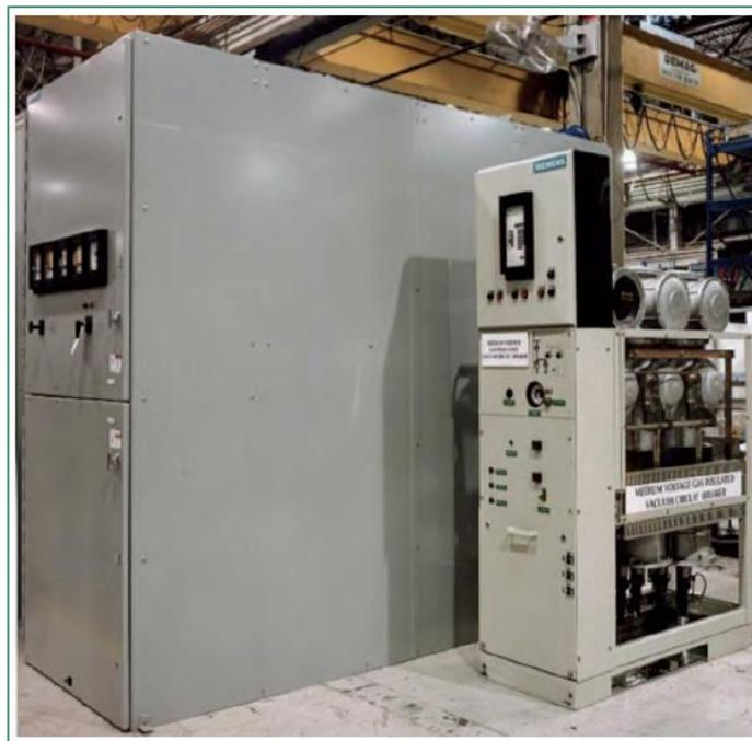
Figure 2-1: 36kV Indoor MV Switchgear comparison (AIS on left, SF<sub>6</sub> on right) [1]
